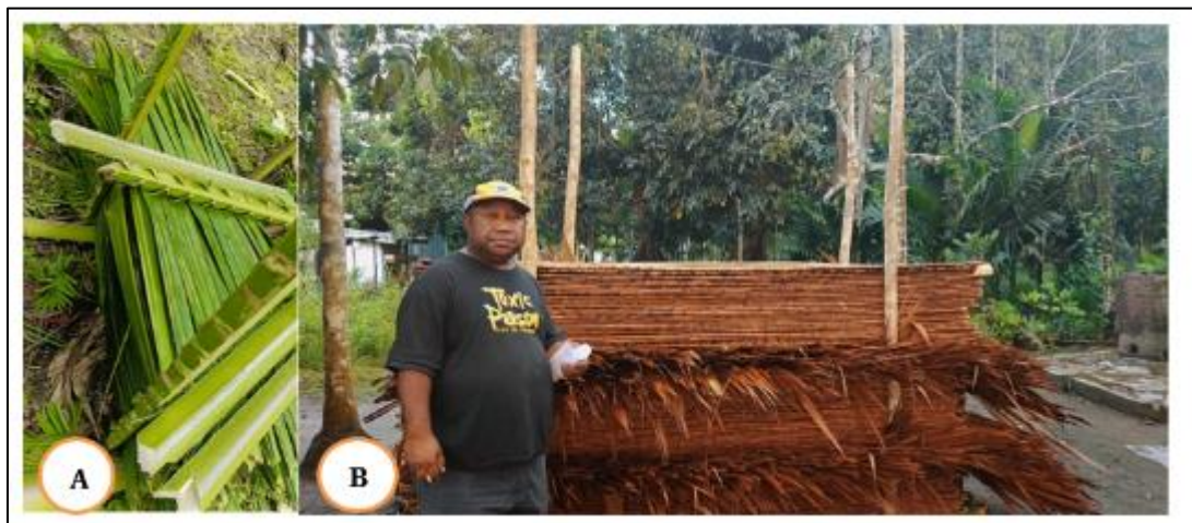
Figure 7 A. Sago palm leaves prepared for roofing; B. Constructed roofing made from sago leaves
