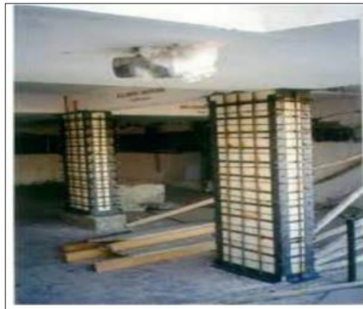
Figure 5 Jacketing of Column
