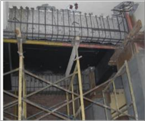
Figure 3 Jacketing of Beam
