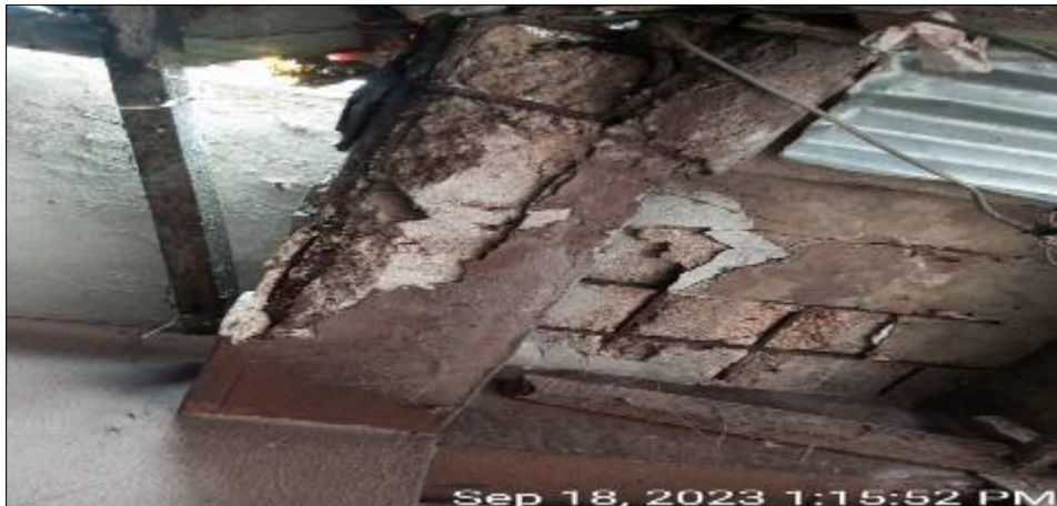
Figure 4 Distressed Building with Concrete Spalling off from Slab and Beam
