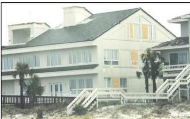
Damage state 2: more than one window but less than the greater of 3 or 20\% of windows
