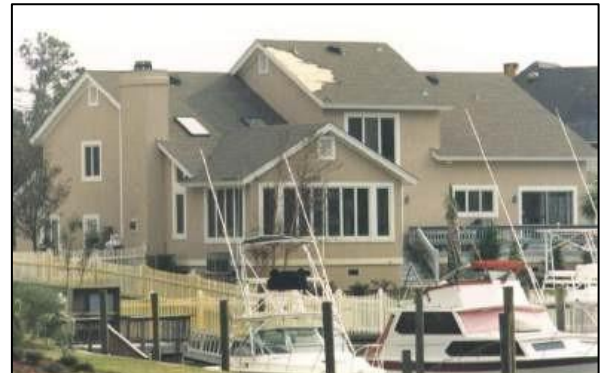
Damage state 1: 2\% - 15\% roof cover loss
