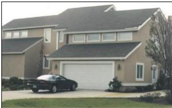
Damage state 0: \leq 2\% roof cover loss
