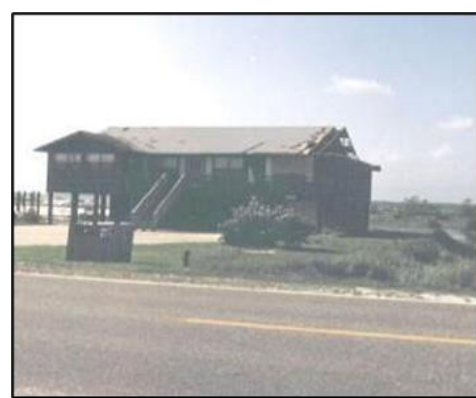
Damage state 3: more than 3 pieces of failed roof sheeting, but less than 15\% panels missing
