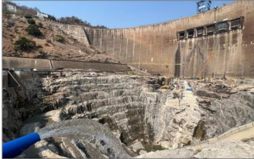
Figure 3 Reshaping of Plunge pool
