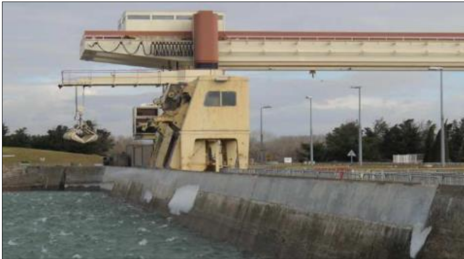
Figure 5 Caderousse Dam's screen rakes after completion of UHPFRC repairs, August 2011 [17]
