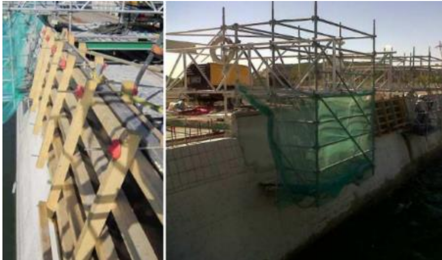
Figure 6 In-situ UHPFRC casting Beaucaire Dam, September 2012 [17]
