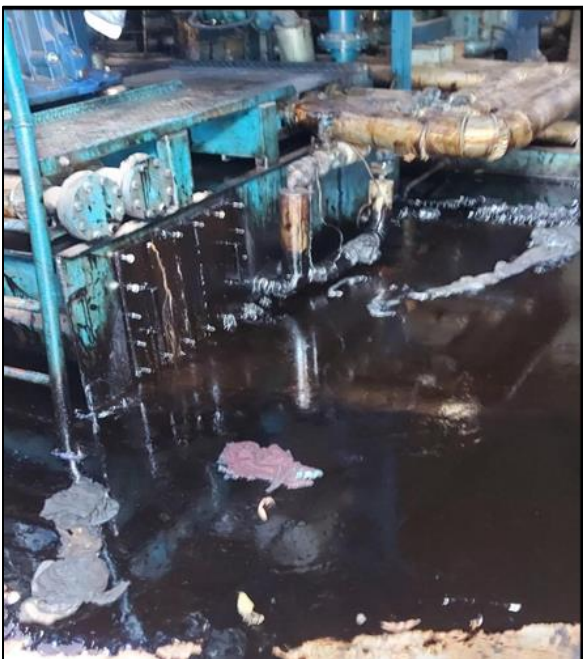
Figure 1 The defective condition of equipment at Kaloum 2 due to lack of maintenance and spare parts
