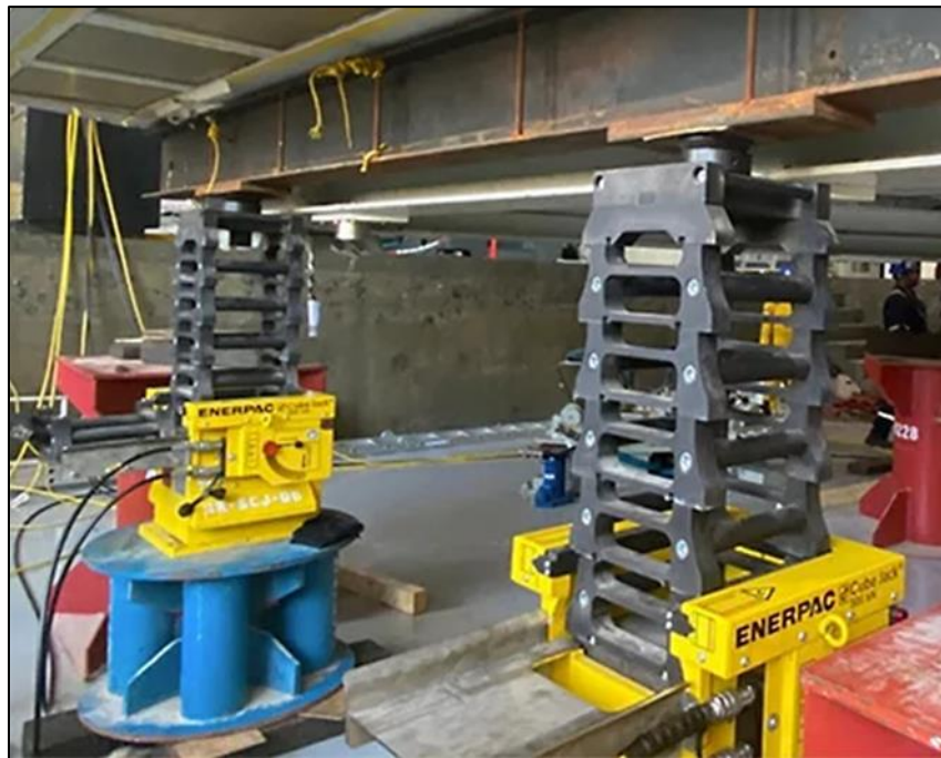
Figure 1 Shows Bridge Jacking System
