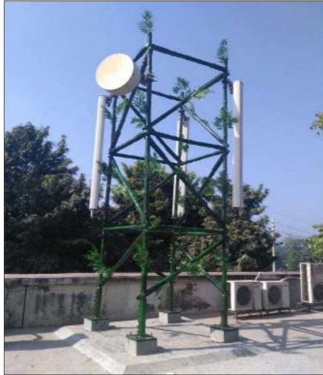
Figure 1 Bamboo tower placed over rooftop at Dhaka, Bangladesh. (Image by Md. Shahrir Alam.) [13]
